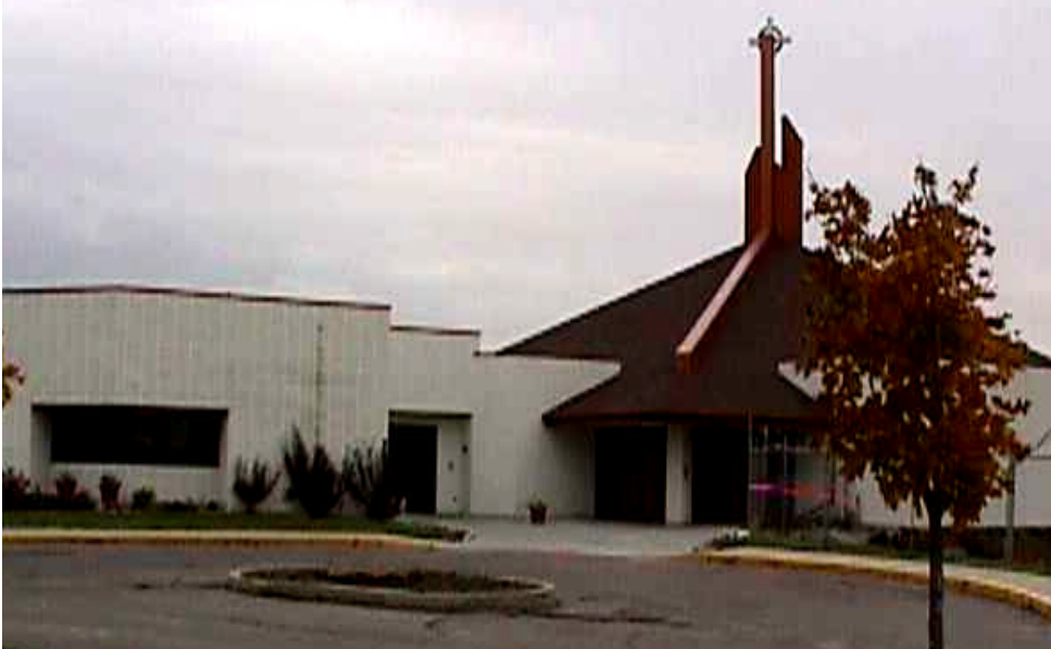
The calm before the construction. New Hope Presbyterian Church will soon be filled with busy construction workers, noisy equipment and tremendous excitement. New Hope is expanding to spread the gospel in Castle Rock, Colorado.
