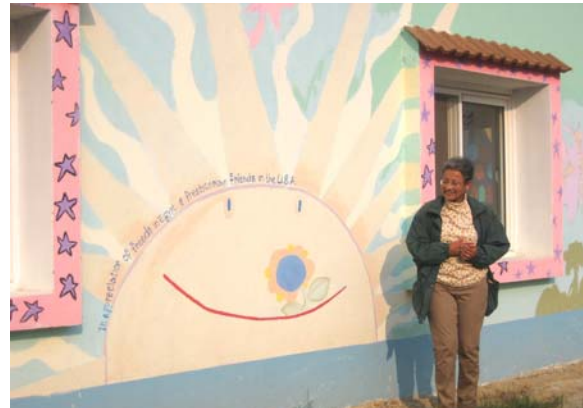
PCUSA Mission Co-Worker Dr. Magda Iskander at one of the buildings of the Health & Hope Oasis, a new facility in Wadi el-Natroun, Egypt, that will provide nutrition assistance and care in a home-like setting for children with cancer and their families. The brightly painted mural says "In appreciation of friends in Egypt and Presbyterian friends in the U.S."
